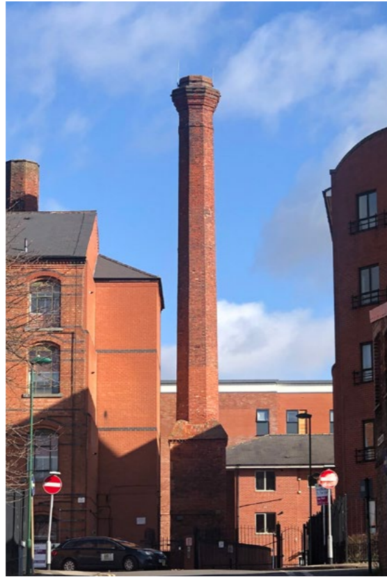
Preserved cotton mill chimneys in Nottingham inspired an octagonal form.
